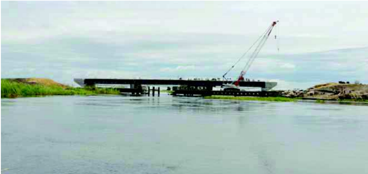
Figure 3: Reconstruction of the bridge on the Mongu-Kalabo Road near Mongu Harbour. The road, linking the districts of Mongu and Kalabo in western Zambia, was extensively damaged during a higher than normal flood event in 2003/2004 season. The road is envisaged to be a gateway between Zambia and Angola for enhanced economic interaction between the two countries. Though the road and bridges are being constructed there is no information on the impact the construction of this road infrastructure will have on flood extent regimes, river channels, silt deposition, or on fish and wildlife movements. This makes it more significant to have in place a flood pattern monitoring system that will facilitate for disaster management preparedness as well as biodiversity monitoring in the wetland (Photograph: Helmschrot, 2015)
