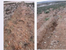
The pipeline at Ratelgat: soil erosion and loss of vegetation cover are visible (Photos: Sophia Etzold)
